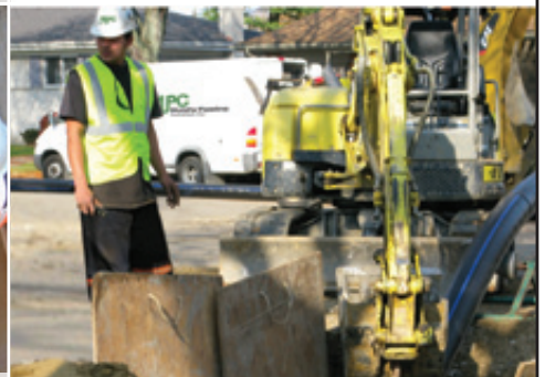
PRE-CHLORINATED PIPE BURSTING
